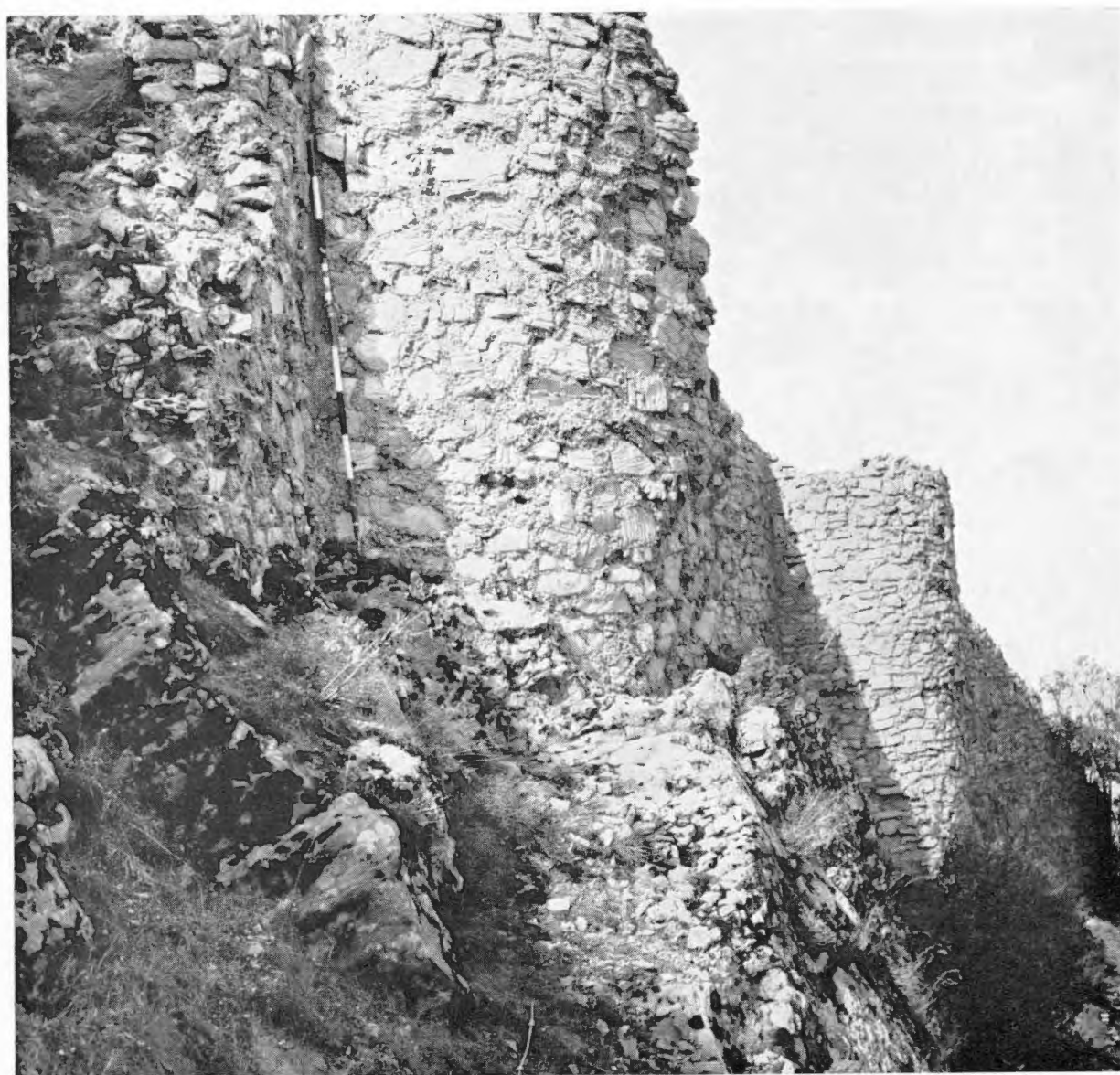
Pl. IIIb. The Upper Castle: buttress towers along the north face.
