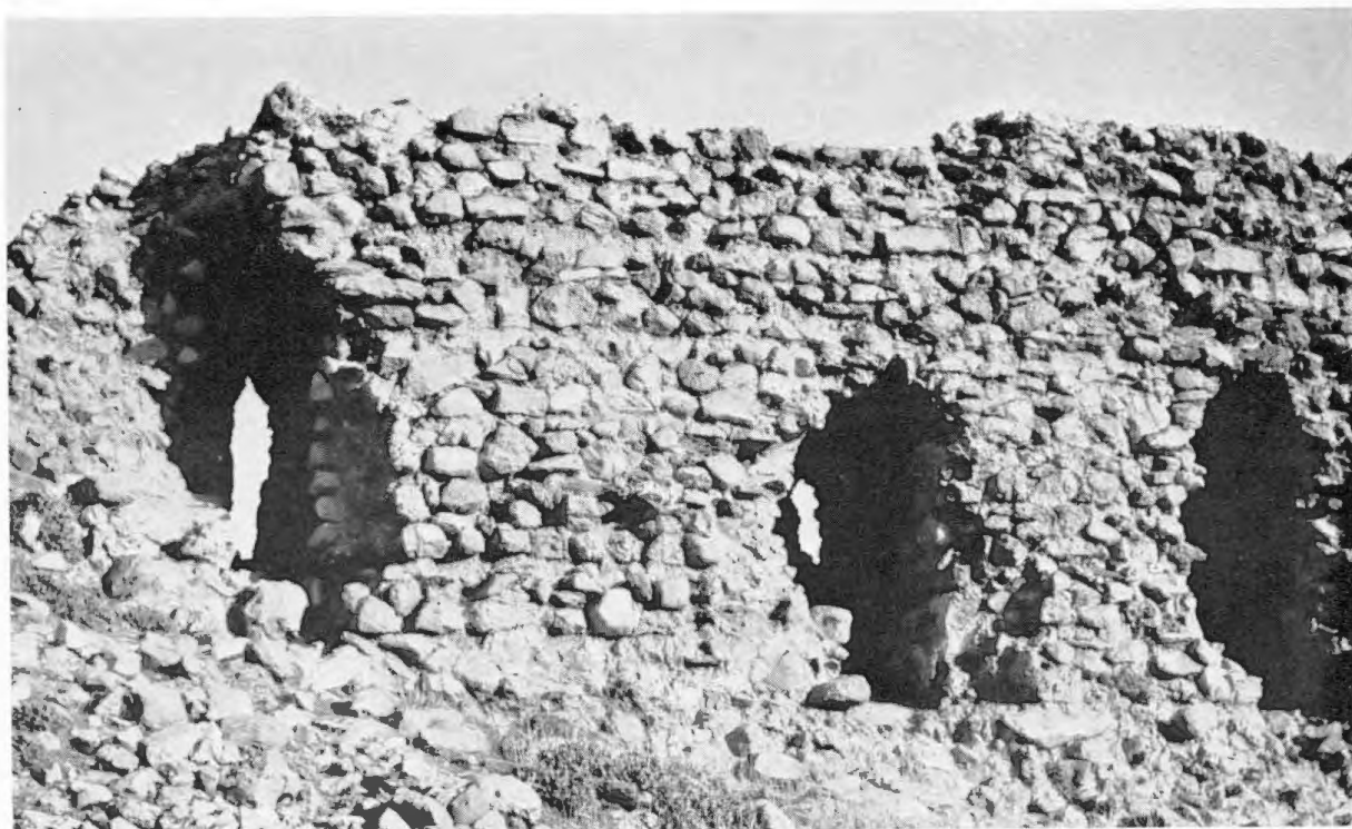
Pl. IIIa. Divar-i Gach: loopholes seen from the inner face of the wall.
