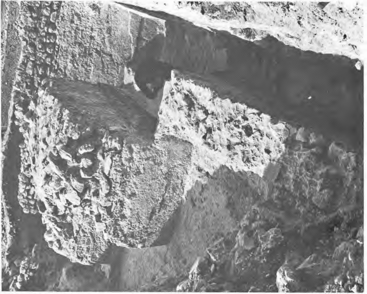
Pl. IVc. L-shaped pier of Kala Dawar chahar taq and blocking wall in corridor.
